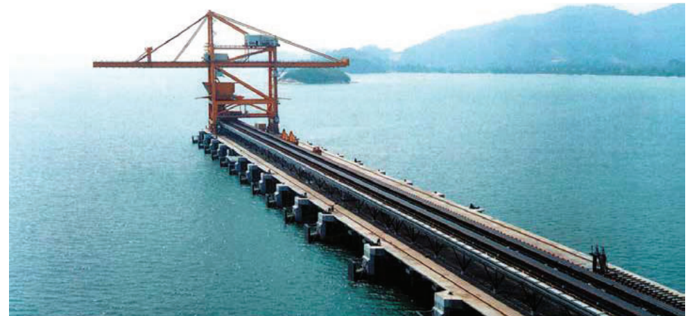
Cross travel of 441.3m, implemented with igus® E4/4 rol e-chain® series 5050R
