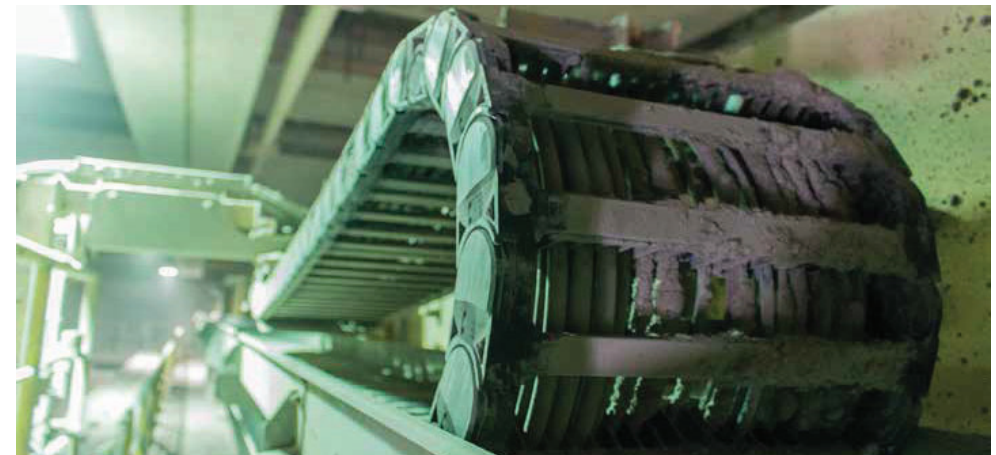
A heavily dust-filled, warm and humid climate pose a great challenge to the components used in this waste bunker.
