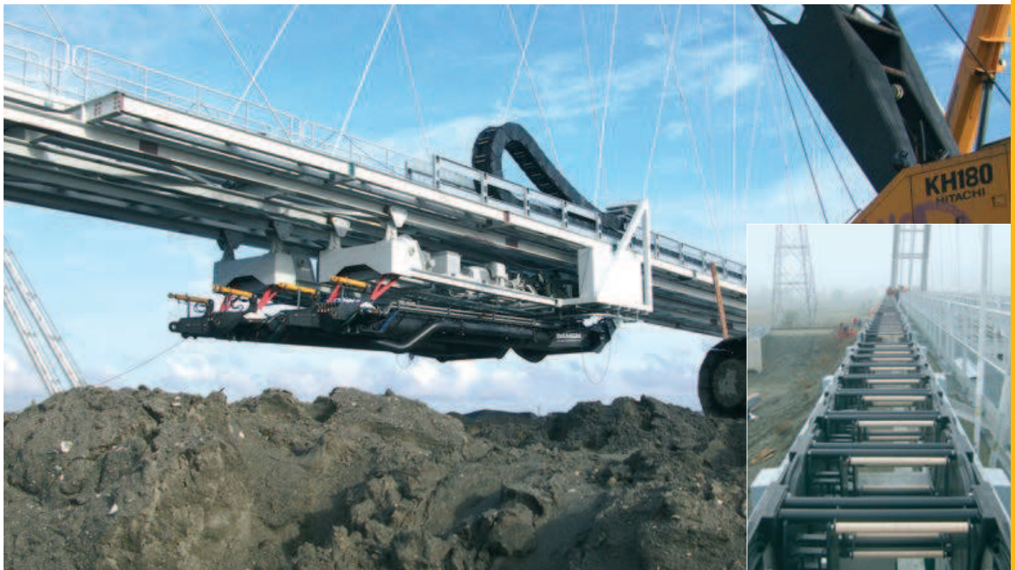
Cleaning of a port basin in Antwerp. On a stroke of 138 meters an e-chain® series E4.350 guides cables and hoses with a total fill weight of 98 kg/m
